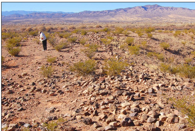
North complex: Looking west along the ridge at the collapsed walls of the main roomblock with about 30 rooms.
