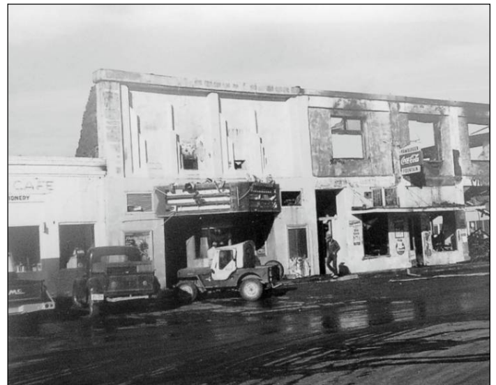
First State Bank collection The empty, burned-out hulks of the buildings are all that remained following the fire. The Park Café, far left, was damaged but survived. The others were razed.
