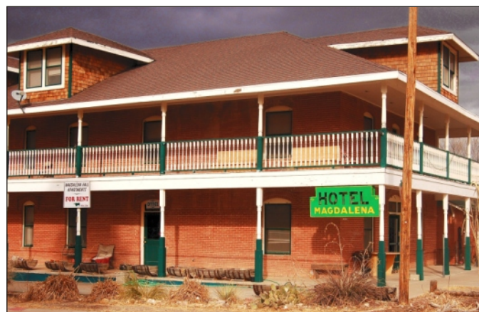
The Magdalena Hotel as it appears today, still offering rooms and monthly apartments. The historic hotel has been renovated several times since the 1929 fire. Most other buildings burned in the fire were never rebuilt.
