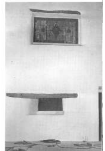
1598 wall after Restoration
