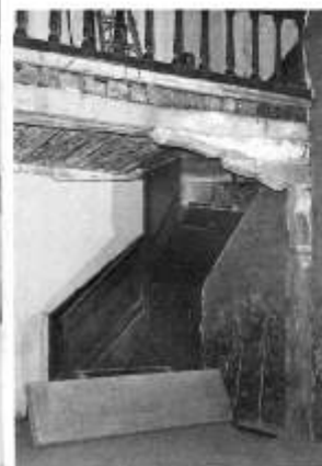
The old staircase
