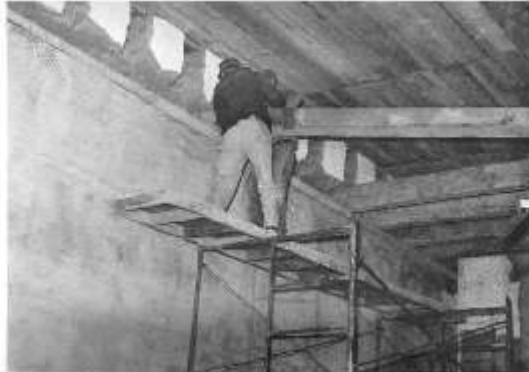
Larry Van Landingham and Vincent Peralta putting vigas in place.
