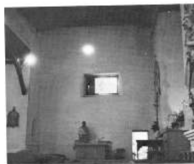
1598 wall before restoration
