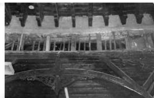
Clerestory window source of original lighting in Sanctuary area.
