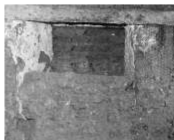
Charred lintels in 1598 door perhaps from 1680 uprising when church was burnt.
