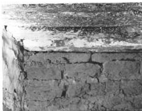
1598 door partially opened showing filled in adobe and yeso.
