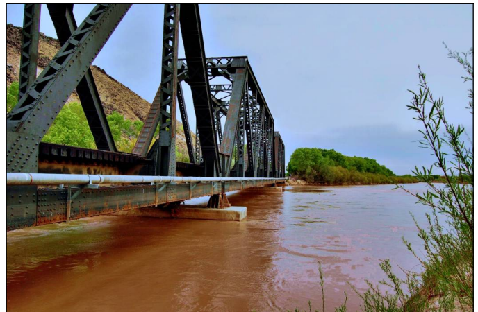
Mainline trestle across the Rio Grande, looking south, the entrance to the Jornada del Muerto and higher ground. Bridge was raised 8 feet after 1929 flood. AT&SF milepost 1005.8
