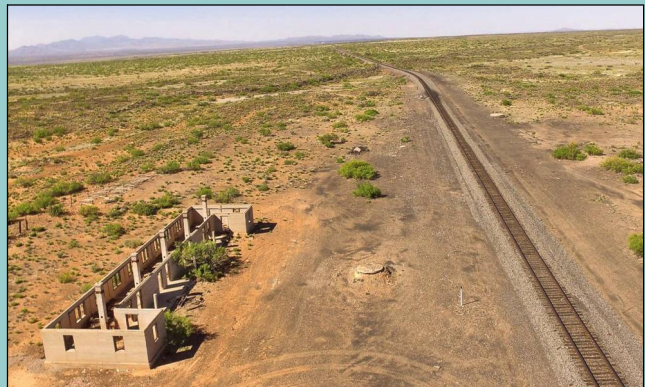
Photo: Paul Harden Drone photo of the Lava Station Section House and water tank foundation, looking north towards San Marcial.
