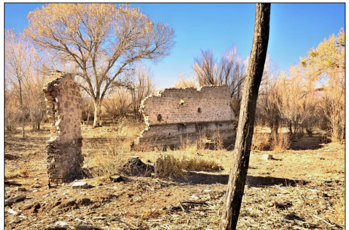
View looking west at Foreman's shack wall (left) and roundhouse wall (center).
