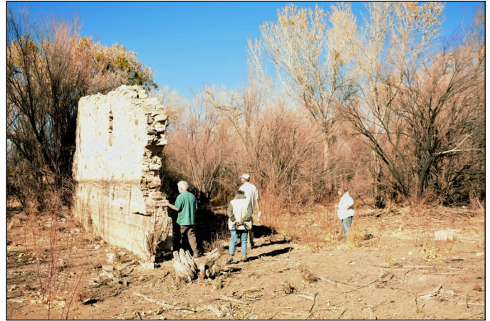
Inspecting the roundhouse wall, looking west. Note water stain on wall, depth of 1929 flood waters.
