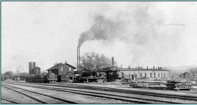
Photo: SCHS, Ralph Lane Collection San Marcial maintenance shops and roundhouse, looking northeast, ca. 1919
