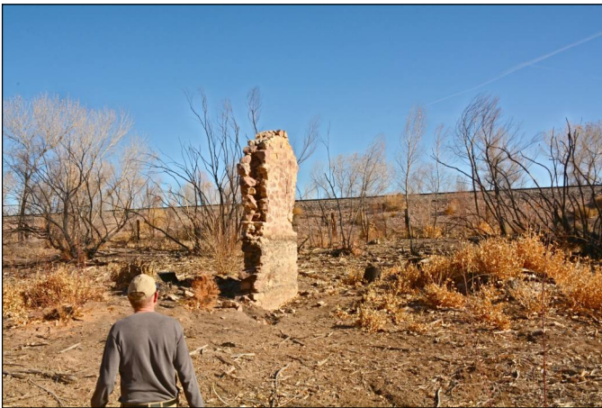
Existing remnant of the back wall of the Foreman's shack, once supporting a pitch roof.
