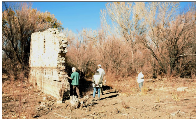
Photo: Paul Harden SCHS members investigating the roundhouse wall on a recent mapping and survey trip to the site. Note water stain on wall showing the 1929 flood depth.
