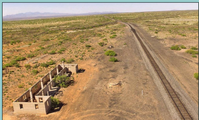
Photo: Paul Harden Drone photo of the Lava Station Section House and water tank foundation, looking north towards San Marcial.
