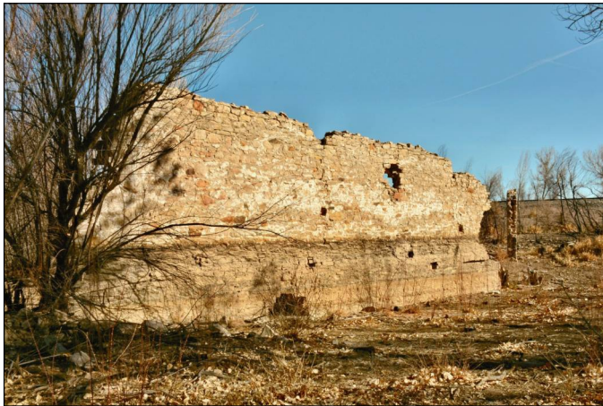
Existing remnant of the roundhouse; northeast wall segment, looking east; turntable to the left
