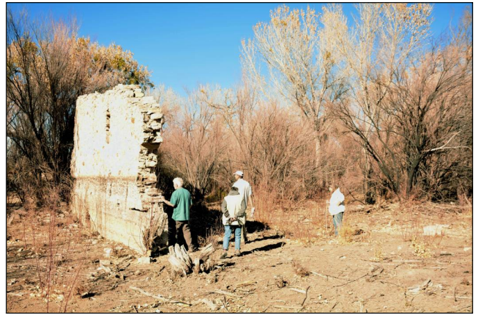
Inspecting the roundhouse wall, looking west. Note water stain on wall, depth of 1929 flood waters.
