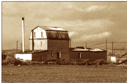
Early photo with the distinctive smoke stack – now gone.
