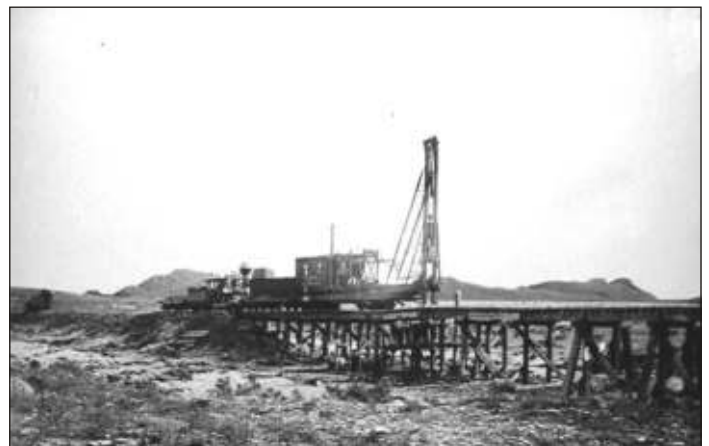
Photo courtesy Socorro County Historical Society Building the Magdalena spur line. This bridge, spanning an arroyo west of the old Water Canyon station, is still visible north of U.S. 60.
